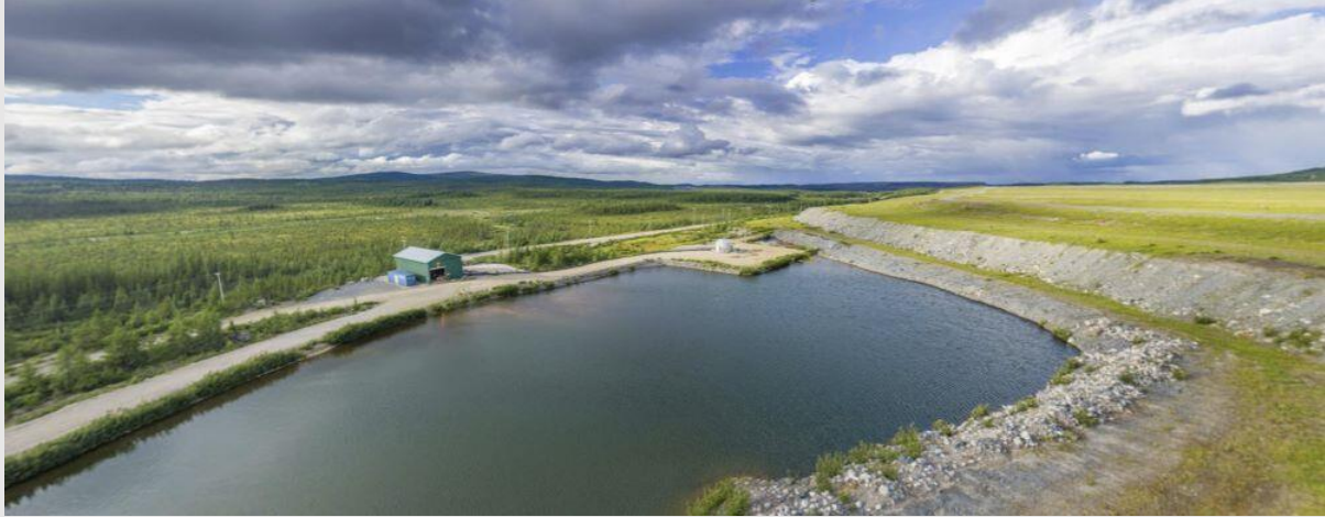
Water treatment and tailings. Courtesy of Troilus Gold Corp.
