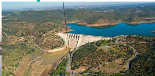
Andevalo Hydroelectric/Water Dam
