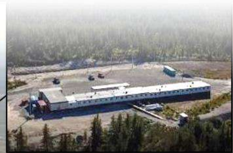
Initial Construction Starter Camp *installed septic
