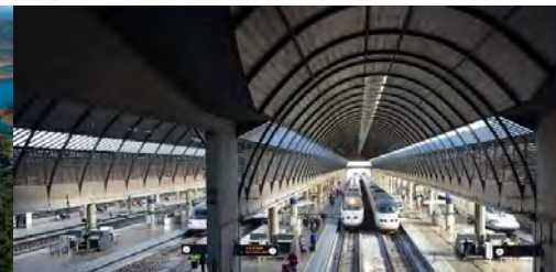
Huelva-Sevilla-Madrid Rail Station
