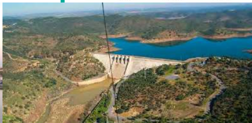
Andevalo Hydroelectric/Water Dam
